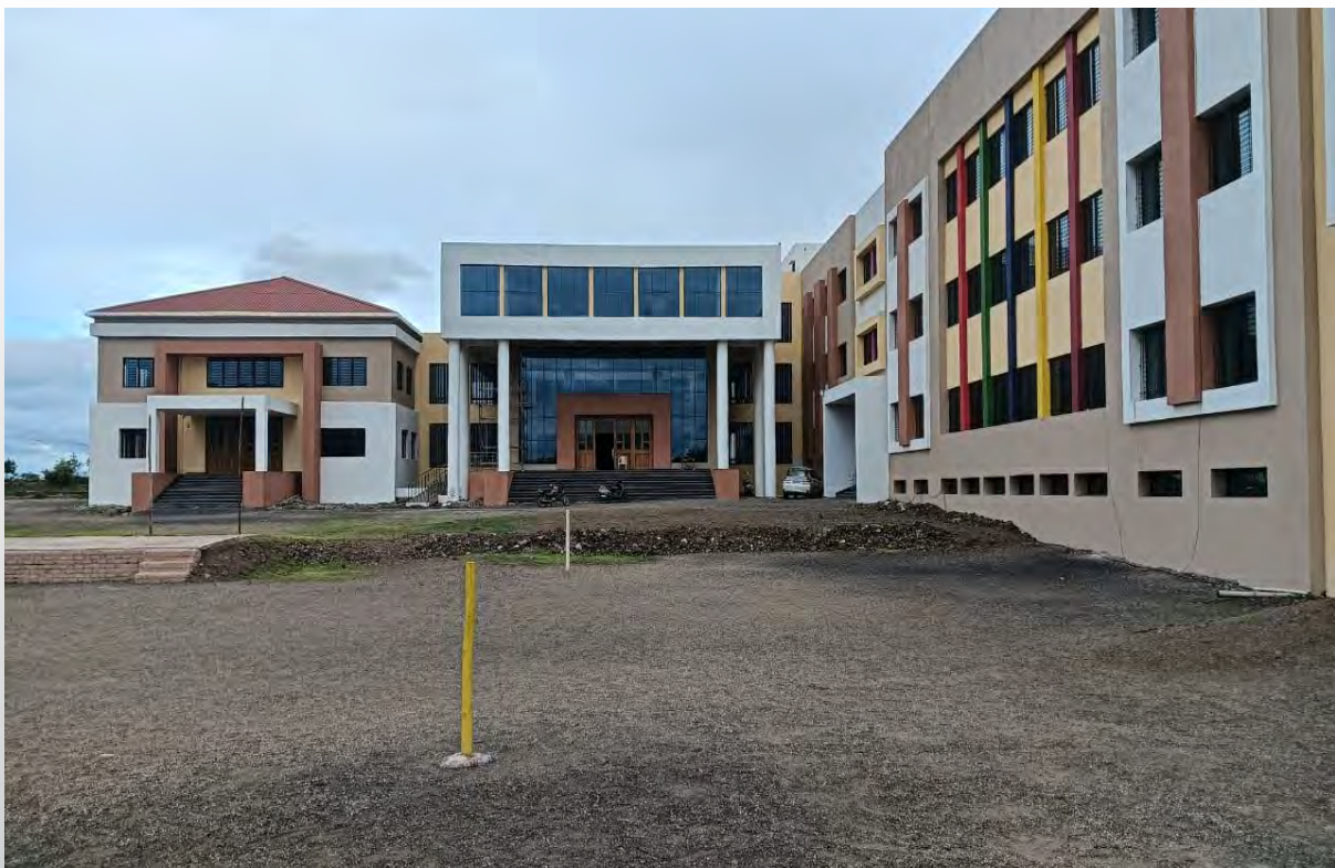
Figure 16- After Construction of new building
