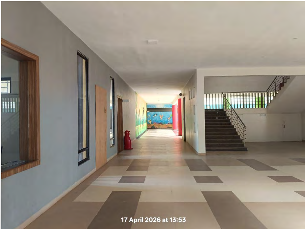
Figure 26- Adequate Natural Light and Ventilation
